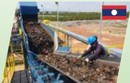
Alternative Fuel Storage and Feeding System, Power Plant Industry
