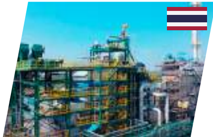
New Green Boiler, Beverage Industry
