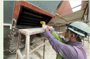
**7. Drive Condition:** Inspect, measure, analyze vibration and measure temperature of the drive system.
