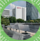
Solar Car Park
