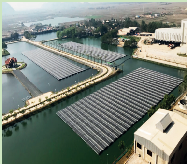
7.0 MW KCC Floating Solar, กทมพช
