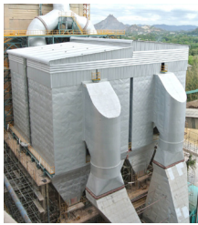
Finish installation of new bag filter
